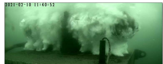
Passive WWS during operation (being air bursted)
